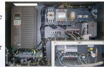
simple drive alternative that is more economical than multi-motor drives. The inverter makes it possible to achieve high extract speeds, which significantly saves energy and time in the drying process.
